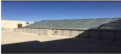
Figure 3: Current skylight at art building.
