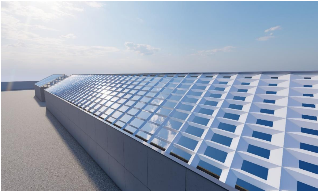
Figure 6: Dynamic louvers passes daylight.
